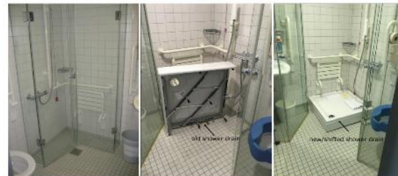
FIG 6 Removable and autoclavable shower insert to prevent direct contact with wastewater. Following unsuccessful eradication and new detections, removable shower tubs were installed to avoid backplash by shifting the shower drain away from the water jet from shower heads.
